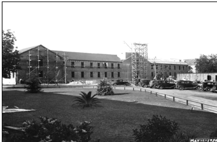
Florida State Hospital (Chattahoochee) benefits from federal construction dollars (1936).
