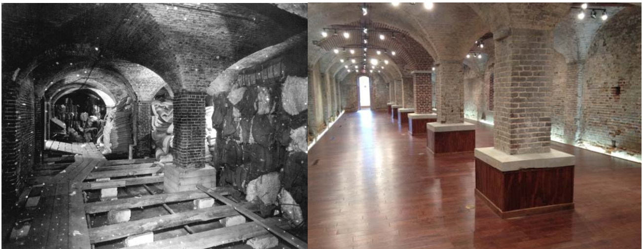
Arsenal Building at Florida State Hospital (Chattahoochee) before and after renovation
