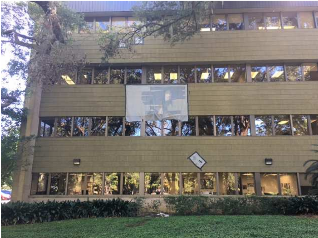
DCF Headquarters at Winewood Office Complex (Tallahassee)
