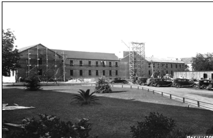
Florida State Hospital (Chattahoochee) benefits from federal construction dollars (1936).
